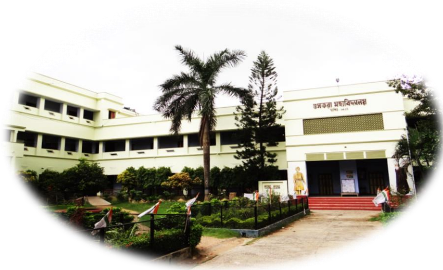
Main Building of the College
